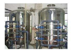
Multimedia Filters are used for removal of sediment and suspended particulate matter. The Multimedia Filter uses a variety of different media types distinctly layered with the coarsest media found on top and the finest at the bottom. This layering of the media allows the larger particles to be removed near the top of the bed while the smaller particles are filtered out toward the bottom.
