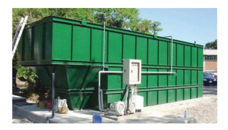
MBBR technology, designed by AAT, employs thousands of polyethylene biofilm carriers operating in mixed motion within an aerated wastewater treatment basin.
