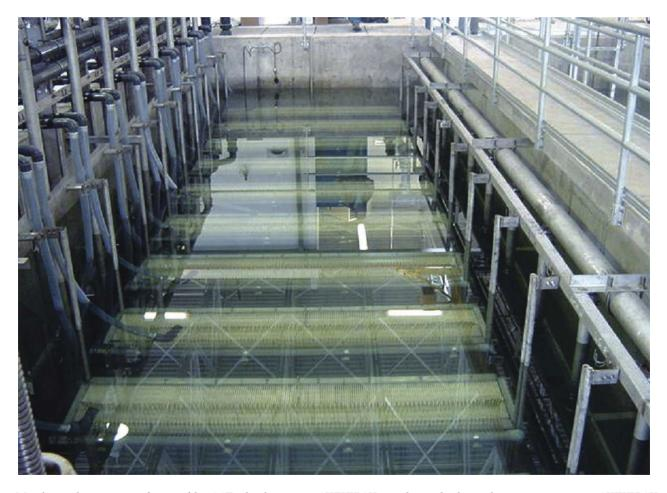
Membrane bioreactors, designed by AAT, also known as AKTIFPAK membrane biological reactor systems or AKTIFPAK -MBRs, comprise a unique wastewater treatment process designed for numerous municipal and industrial applications. Membrane bioreactor systems may be used in such applications as water reuse, new housing developments, parks and resorts, retrofits, and turnkey projects.
