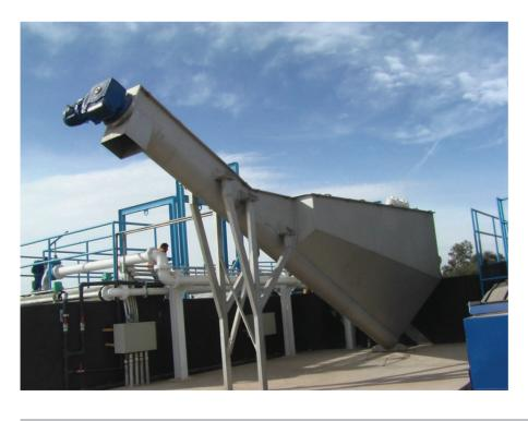
Grit classifiers are used to separate / dewater the sucked grit and the water content. Waste containers are placed just under the discharge chute of the classifier.
