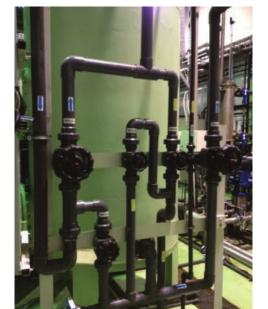
The raw water is passed through Cation Unit and then through the Anion Unit. The Total ionic load gets absorbed on resin, and you get water with Total Dissolved Solids (TDS).
