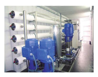
What the membrane surface keeps always clear and unblocked is the "cross flow" action realizing within membrane element. While a part of liquid (product water) passes through membrane due to the cross flow another part of liquid (concentrated water) hiders bonding impurities to membrane. Surface of the membrane is swept by an auto flush application periodically to keep clean membrane.
